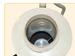
View Down Top Outlet
