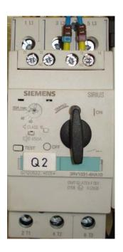
\*\*\* Thermic may be blown. If it is blown, you should turn it in its normal position.
