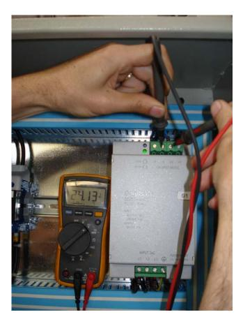
\*\*\* You need to check **''G1'' DC** power supply in beam box for its input and output voltages. You should check if there is **24V DC** in output of power supply. When the gauger is on **DC**, one side of it should be on no.2 point of **G1** and the other side should be on no.11 cable. If you gauge **24V DC** check the things below.
